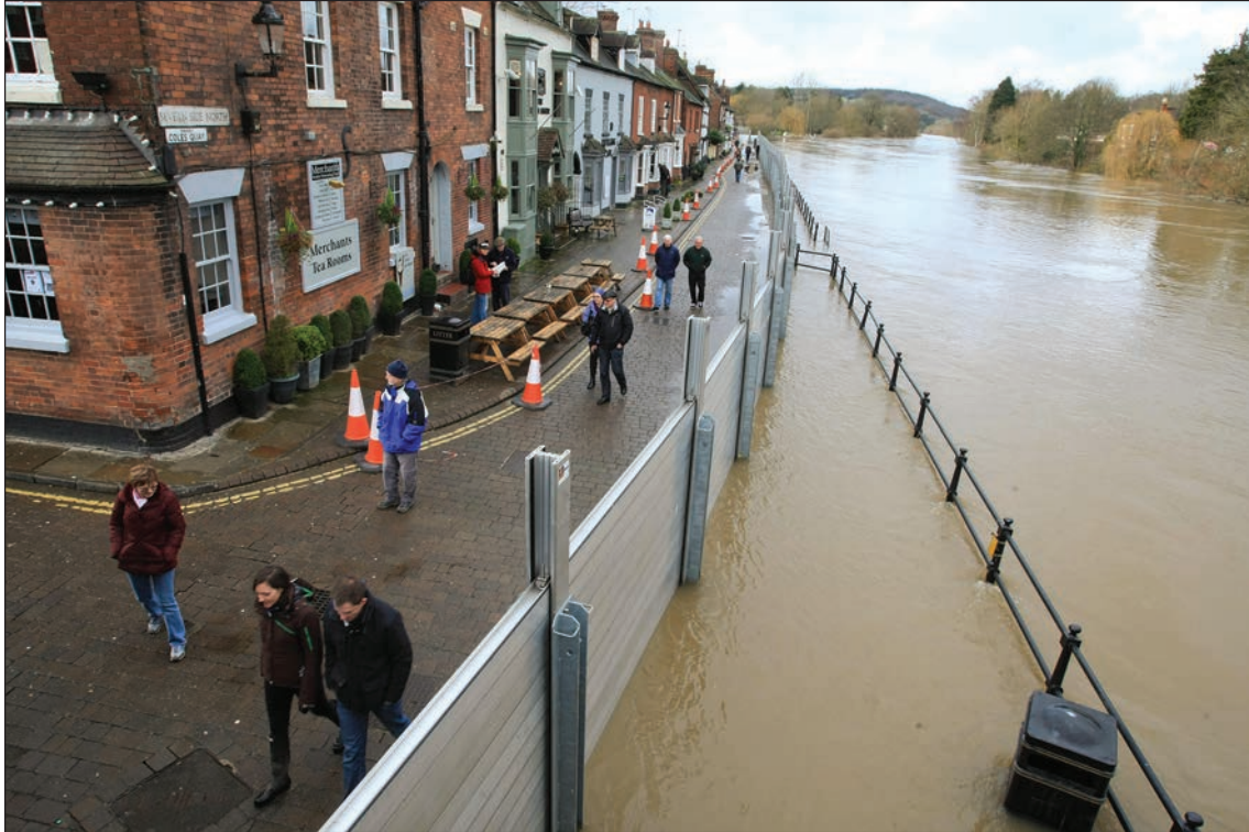
Photograph 2.1 - A flood event in Bewdley
