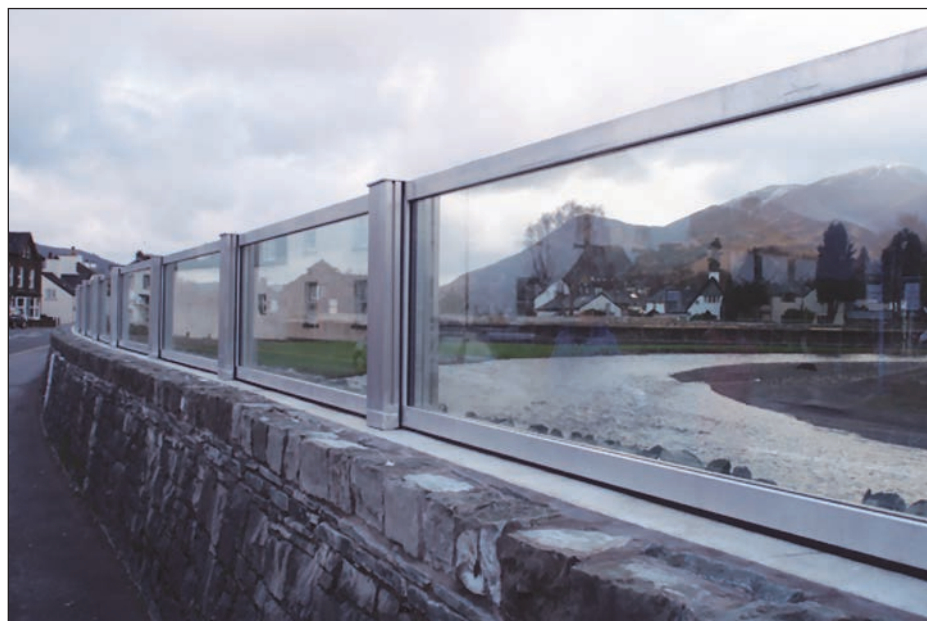
Photograph 3.4 - An example of flood defences on the River Derwent in Keswick
